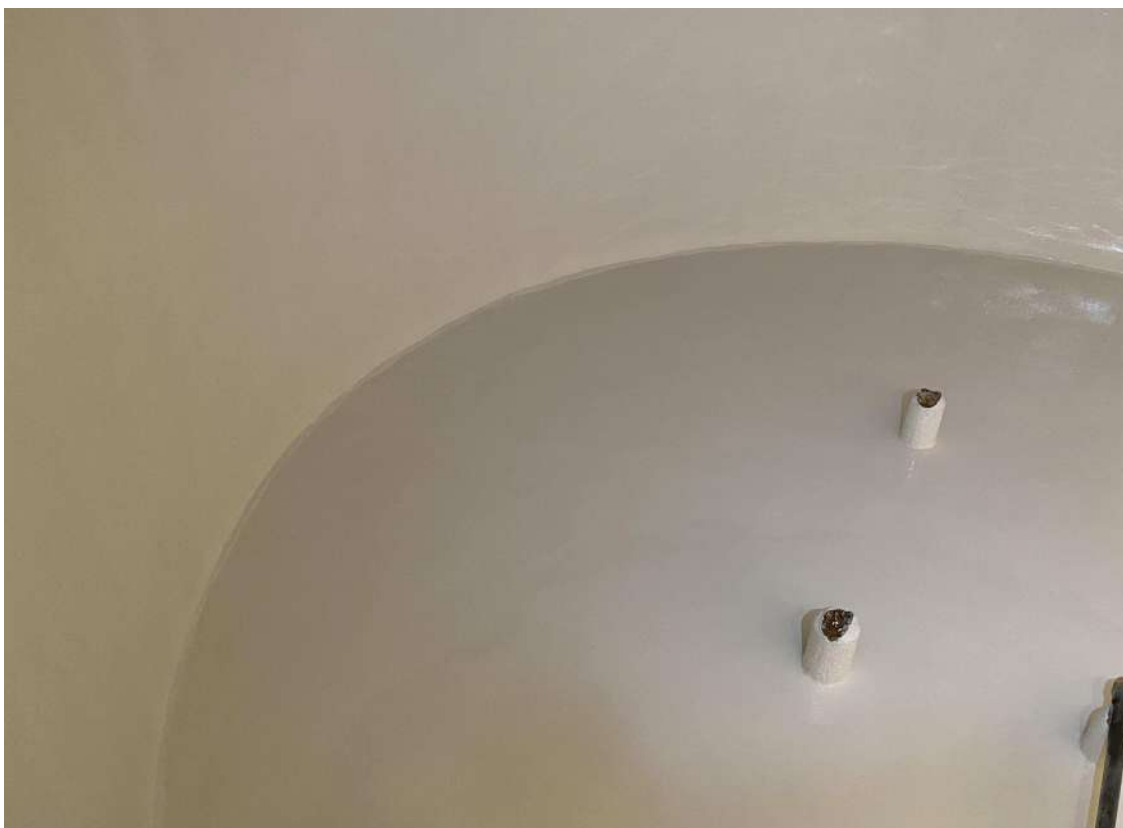
Coating of a water tank in SOUPLETHANE WP, March 2020
