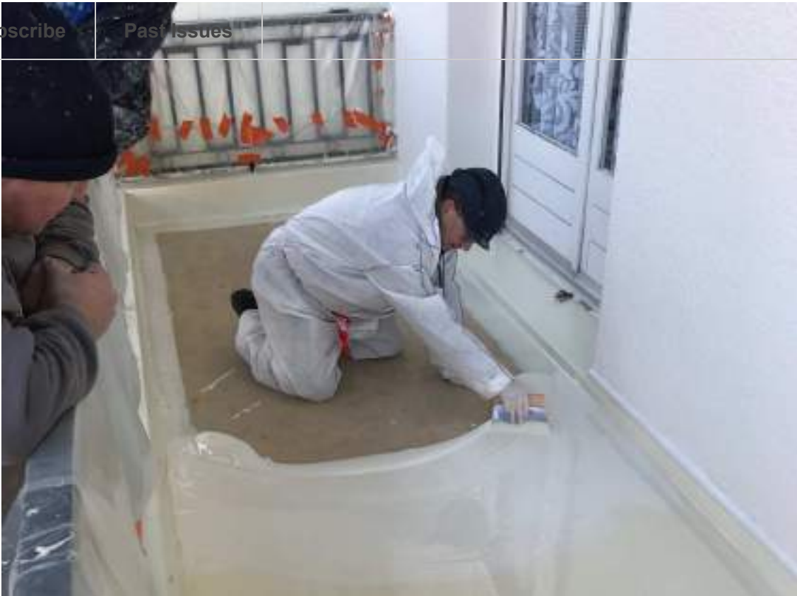
Application on balcony, Souplethane 5
