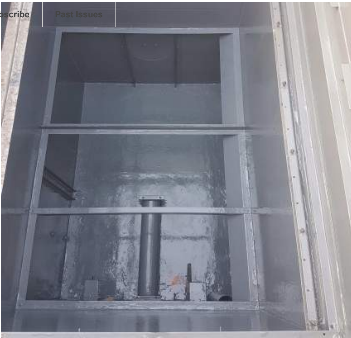
Rehabilitation of a cooling tower interior
