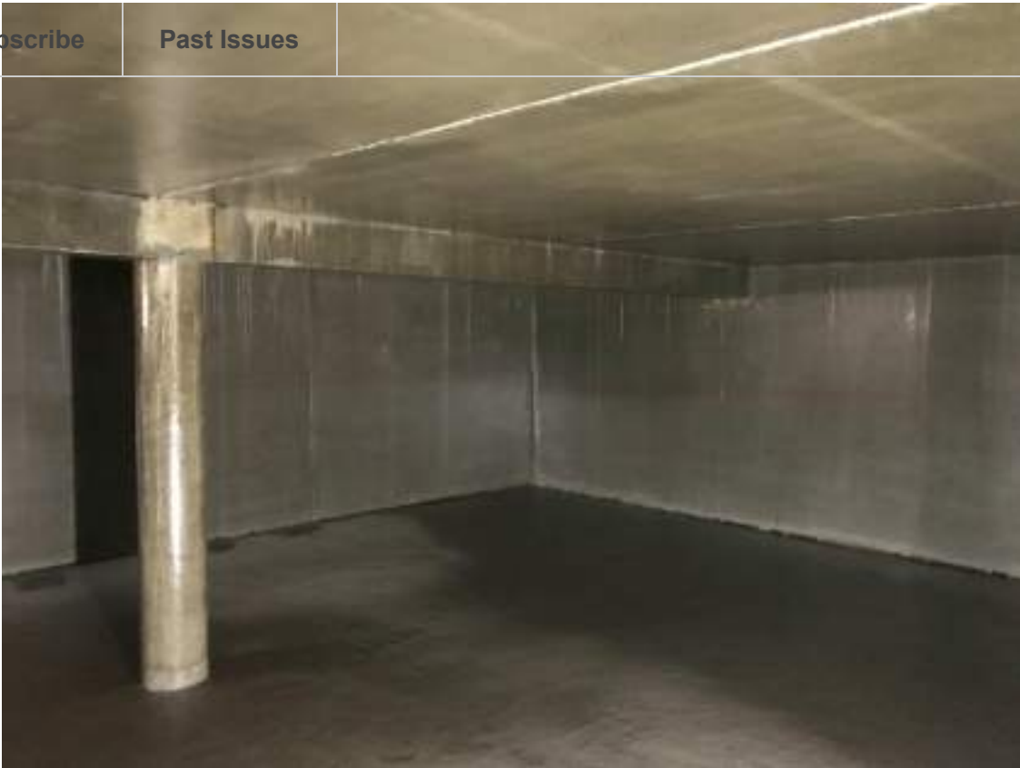
Floor, wall and ceiling, Souplethane 5, PU Aqueux
