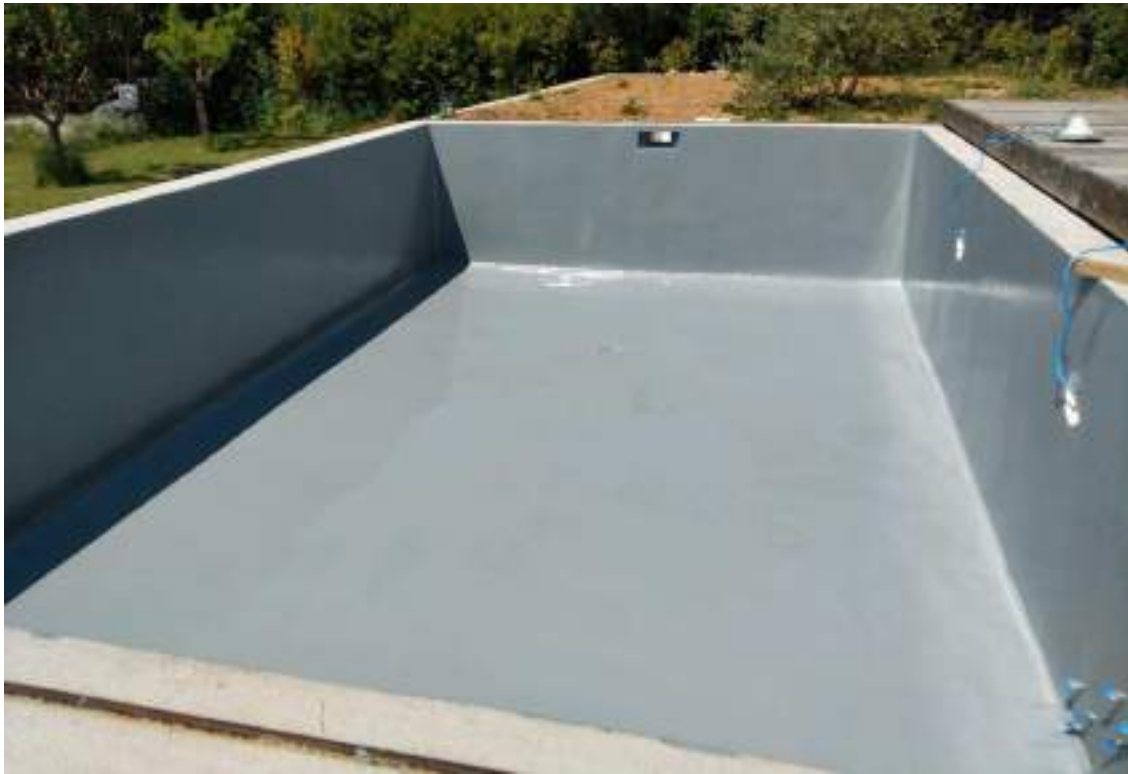
Swimming pool renovation, Souplethane Floor
