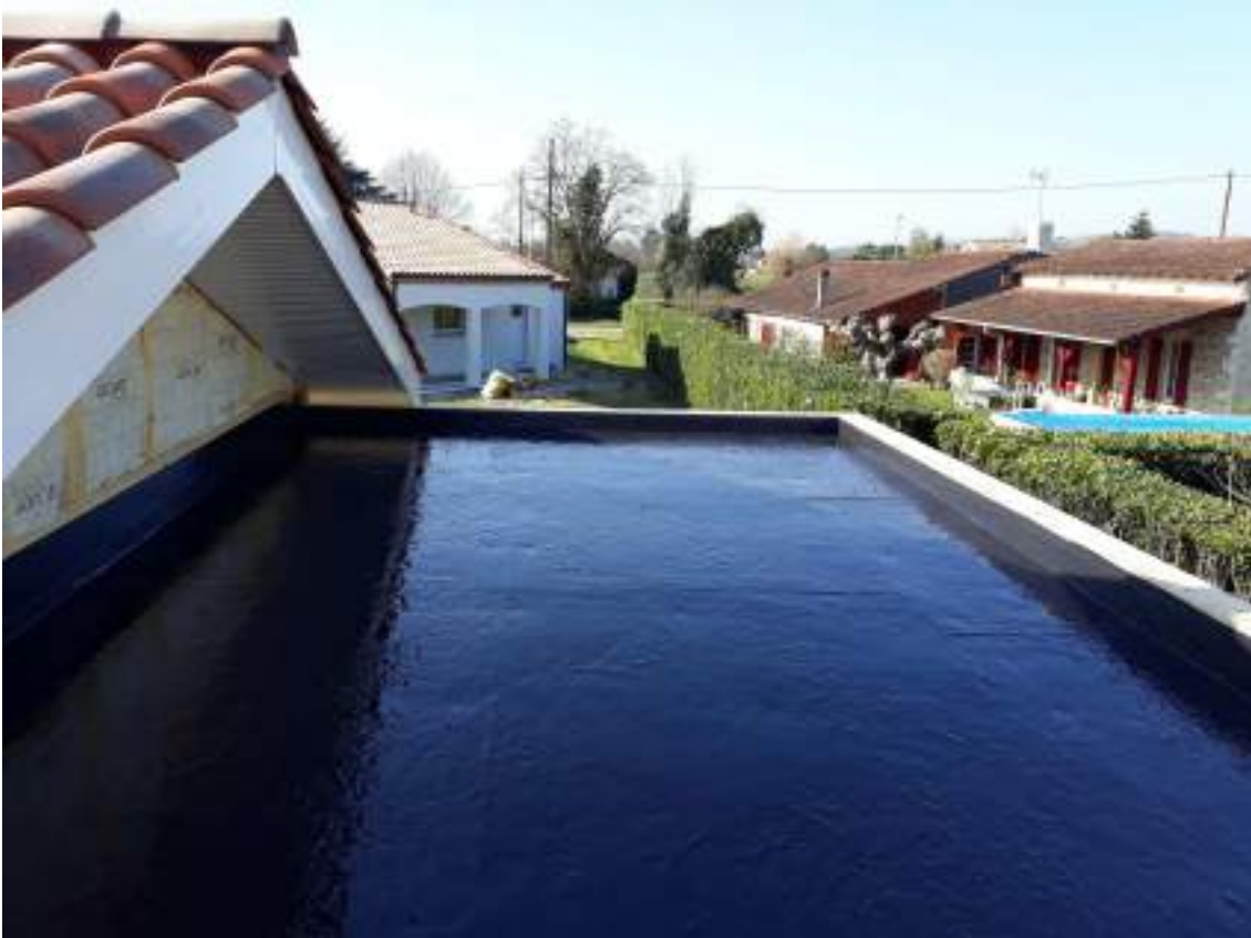
Black Souplethane 5 application on wooden terrace
