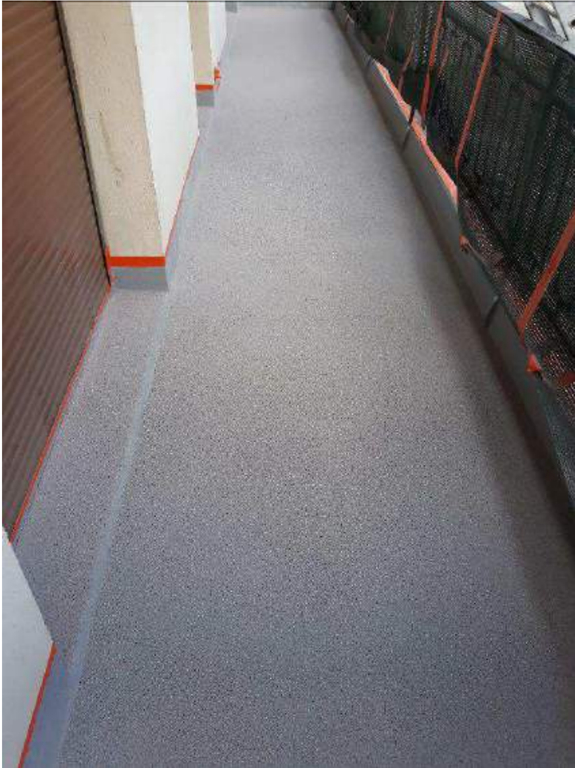
Souplethane 5, Kemipox, Poudrec and ASPIC 7035 application on balcony
