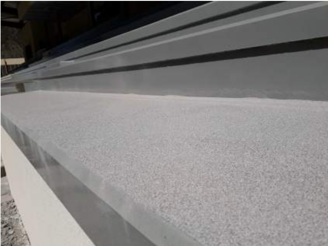
Souplethane 5 application and Poudrec finish on stone bleachers
